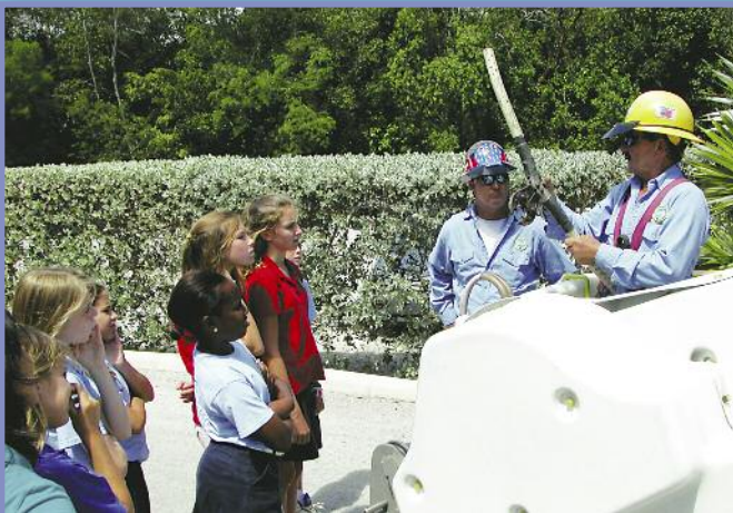
Linemen Gene Ehrenkauffer (in bucket) and Andy Baxter show students from the Academy the tools and equipment used by linemen when working on power lines.
